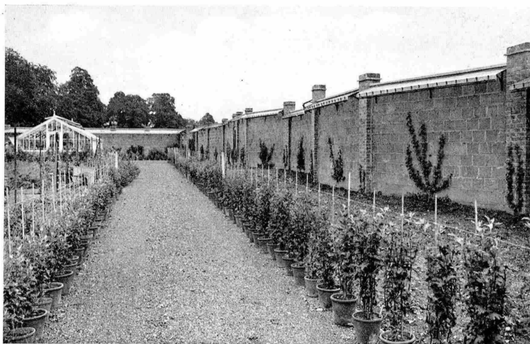
Copyright. 11.—VIEW IN KITCHEN GARDEN. "COUNTRY LIFE." Showing a new use of hollow bricks for the enclosing walls.
